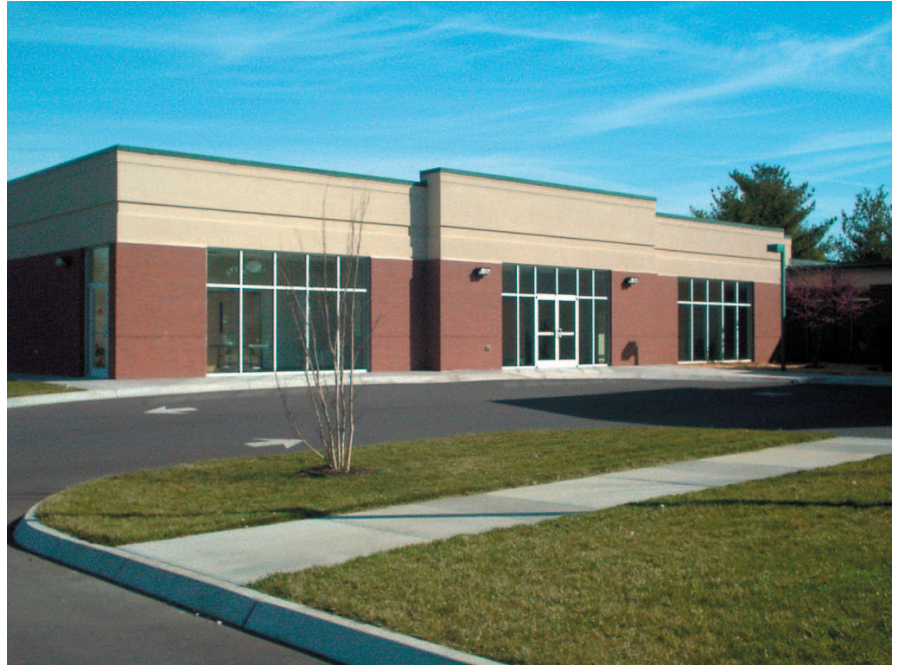
John T. O'Conner Senior Center Addition
