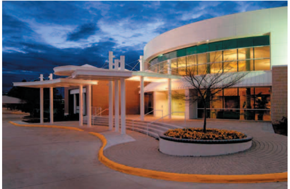
Green Clinic Surgical Hospital in Ruston, Louisiana
